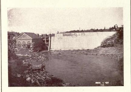
N extended view showing power house and completed rollway looking upstream. The water is coming through the dam in the first two sections of the bulkhead and work is now proceeding on the bulkhead and on the canal.
